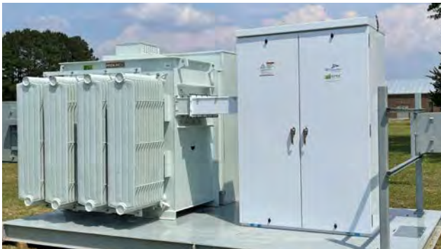
PV UNIT SUBSTATION
